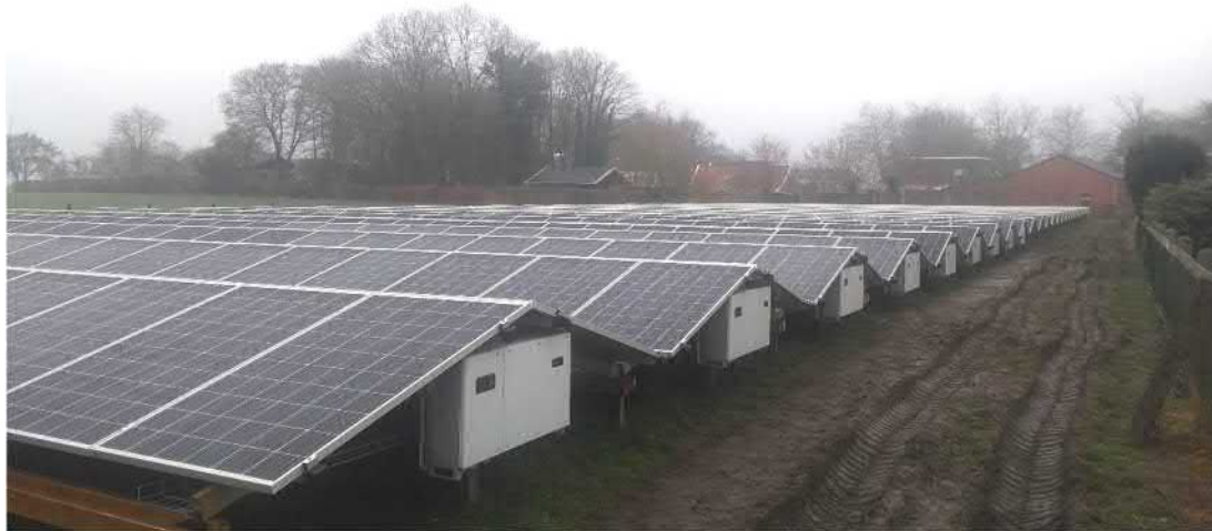
Photo 1-4: Solar panels with east-west facing configuration (image reproduced courtesy of Huawei)
