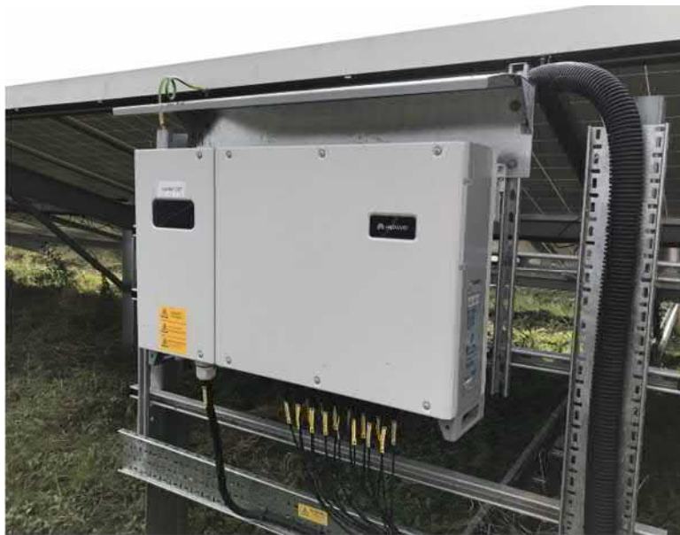
Photo 1-8: Typical string inverter (image reproduced courtesy of Huawei)
