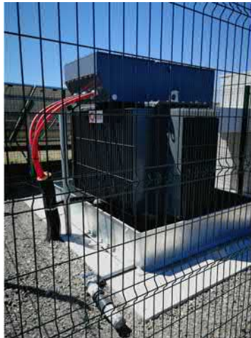
Photo 1-10: Typical outdoor transformer
